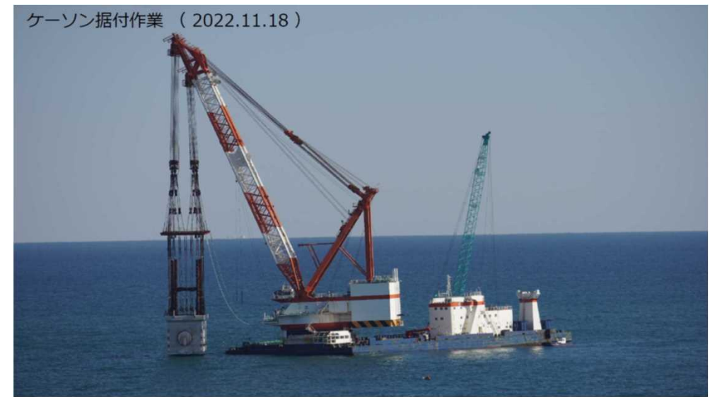
Construction progress: caisson installation on 18 Nov 2022 Source: TEPCO's material on 19 Dec 2022
