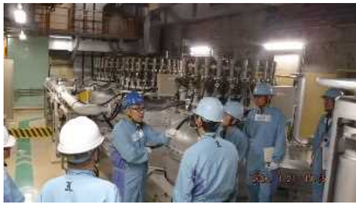
Photo2-1 Trial operation of new inspection program (Tomari NPS, January 21, 2019)
