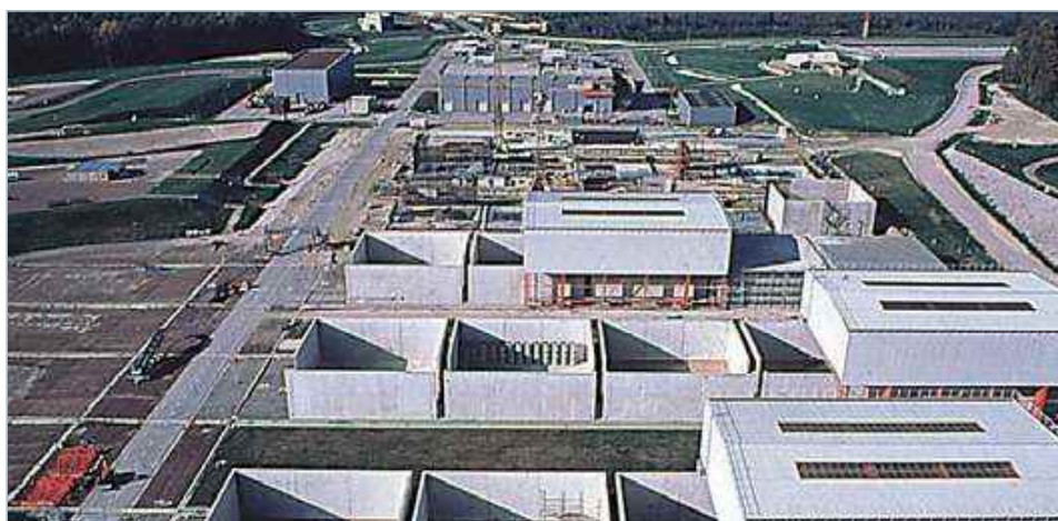
At Andra's CSA disposal facility (Aube), waste packages are placed in concrete cells or "disposal structures". When they are full, the cells are covered with a concrete slab and polyurethane membrane.
