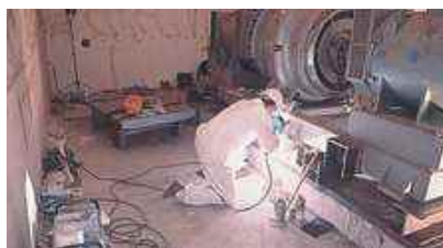
Decommissioning operations (VLLW).
