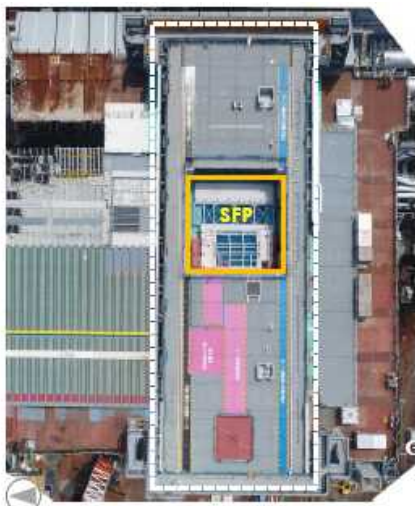
Top view of Unit 3 reactor building before installation of domed cover (As of July 2017) (Photo provided by TEPCO)
