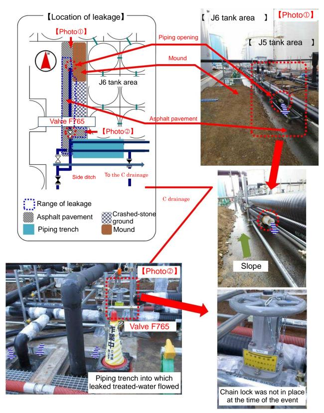
Figure 3. Situation of leakage on site\*5
