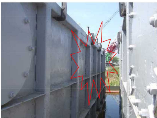
Photograph 3 Leaking portion
