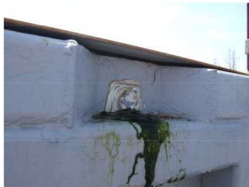
Photograph 2 Leaking portion
