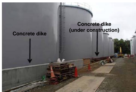
Figure 10 Situation of further height raising of dike *2 (J1 area)
