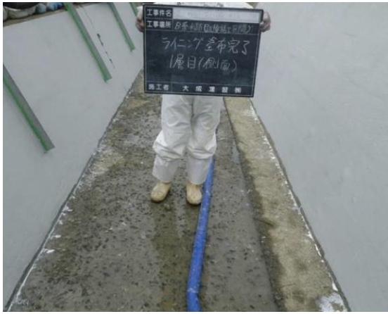
Figure 12 Situation of B drainage ditch lining *2
