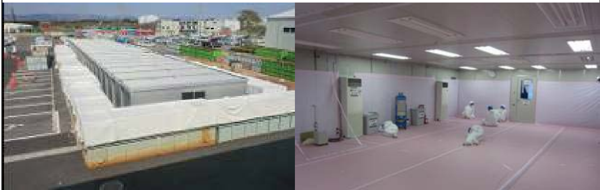
Exterior (left) and interior (right) appearances of on-site rest stations
