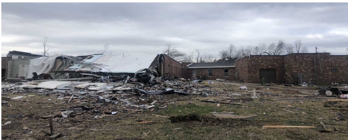
Figure 6.4.6. Damage to one wing of the Mayfield Health and Rehabilitation Center (Image acquired by the FAST).
