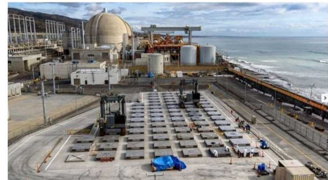
The dry used fuel storage facility at the San Onofre plant in California (Image: Southern California Edison)
