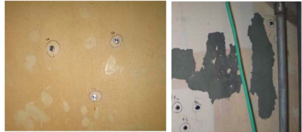
Test Area – As Found with Dollies Installed
