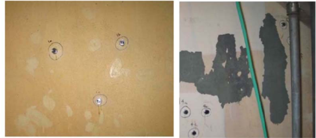
Test Area - As Found with Dollies Installed
