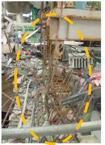
Photographed by TEPCO on October 5, 2011 <u>Floor damage in the southwest area of the 5th floor</u> (upward-vent reinforcing bars)
