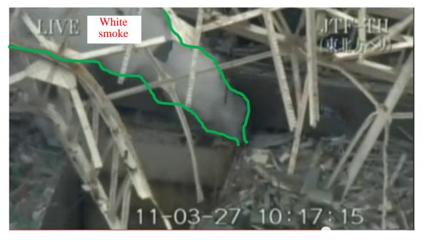
Figure 6.4 White Smoke rising from the Reactor Building of Unit 3 (site 2) Source: Abstracted by the NRA from video images taken by the Ministry of Defense (on March 27, 2011) and disclosed on the same day
