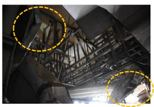
Photographed by the NRA on July 12, 2013 Ceiling damage in the northwest area of the 3rd floor (duct damage)
