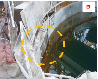
Deformation of the exhaust port net of the exhaust duct above the reactor well on the 5th floor (deformed outward) (photographed by TEPCO on November 8, 2011)
