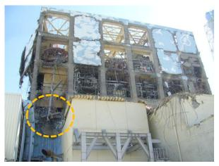
Photographed by TEPCO on March 18, 2011 Complete destruction of the wall west of the staircase in the northwest area of the 3rd floor
