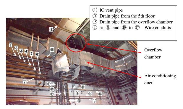
Figure 3.6 Pipe Layout near a Location where Water was seen coming out
