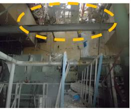
Photographed by TEPCO on November 8, 2011 Ceiling damage in the southwest area of the 4th floor
