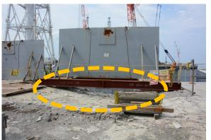
Photographed by the NRA on July 11, 2013 Downward deformation in the north area of the 5th floor
