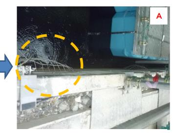
Deformation of the exhaust port net of the exhaust duct above the SFP on the 5th floor (deformed outward) (photographed by TEPCO on November 8, 2011)
