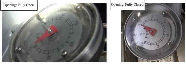
Photographed by the NRA on May 31, 2013. <IC system "A" (2A) opening meter>
