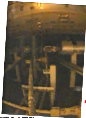
主蒸気配管Cの下側
