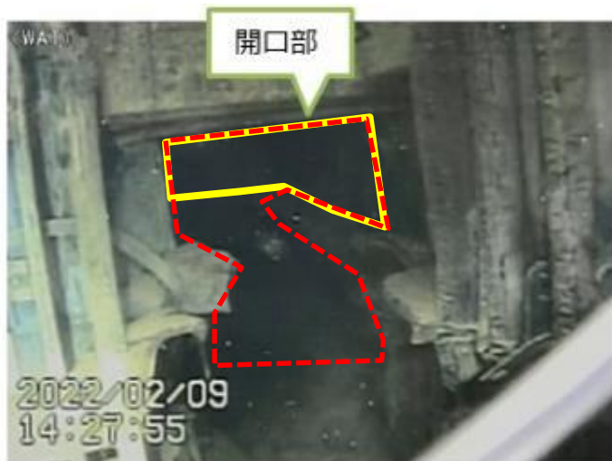
ペDESTAL開口部俯瞰
