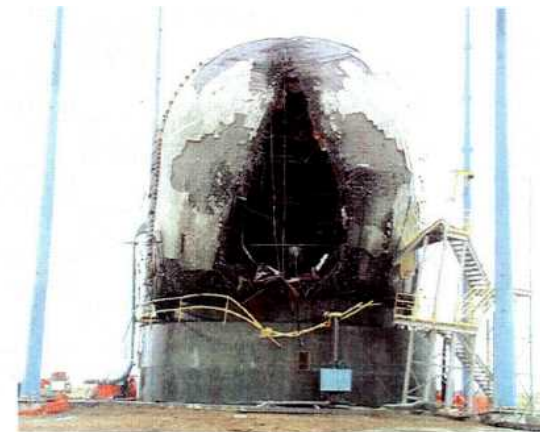
Figure 63 PCCV Model after the Structural Failure Mode Test
