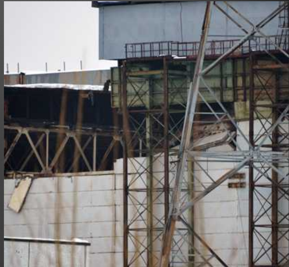
Collapsed portion of Chernobyl sarcophagus roof
