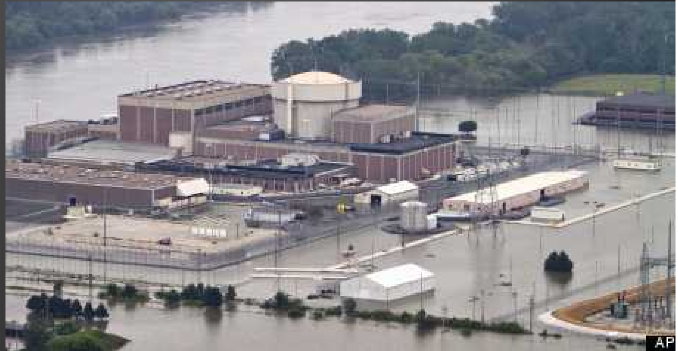
Ft Calhoun Nuclear Power Plant, Nebraska, US, June, 2011
